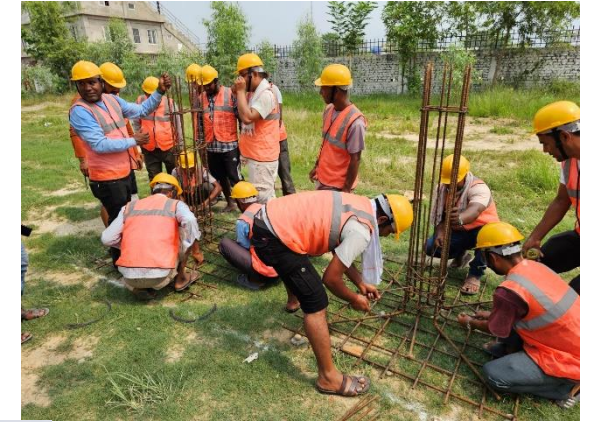
Setting up Footing
